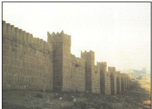
Looking west along the restored northern outer wall of Nineveh toward the Nergal Gate in the distance. The circuit of the walls of Nineveh is about 12 km. [source: Cultural Atlas of Mesopotamia by Michael Roaf].
